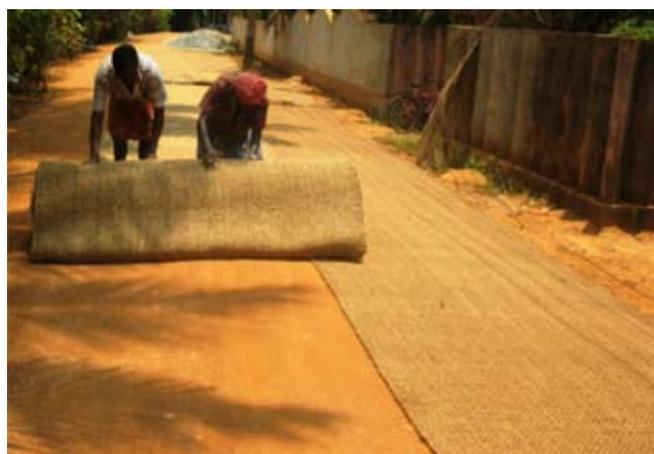
**Fig. 21** : Another view of a road during constructions**Table 8** : Properties of coir geotextile
